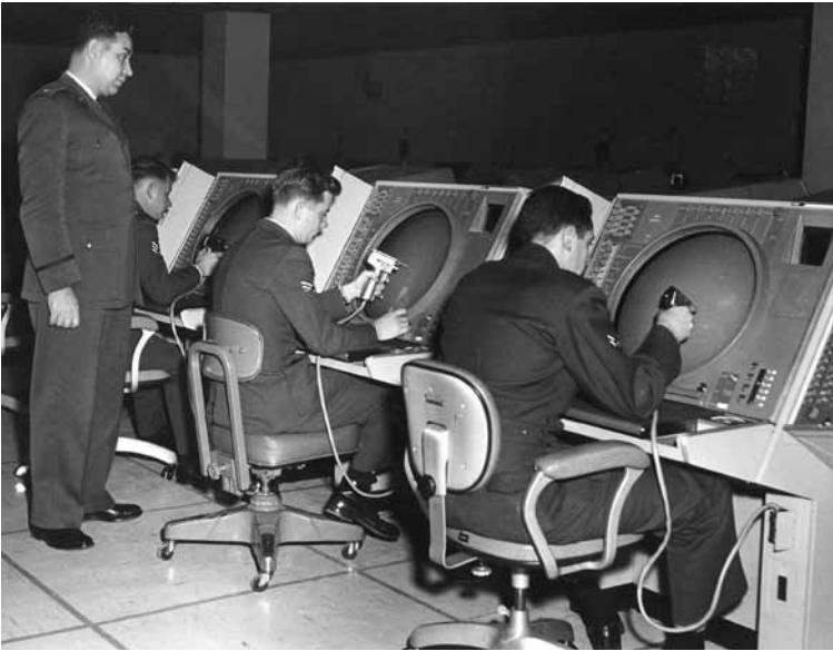
Abb. 5 SAGE Lightgun Interface, 1950 2
